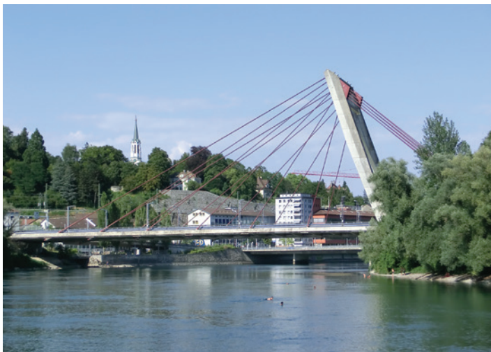
Bridge over the Rhine in Schaffhausen
