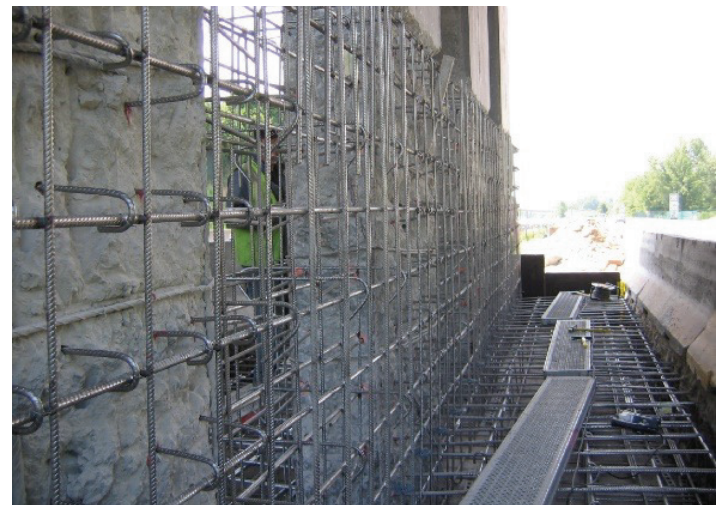
Repair of the central pier of a highway bridge
