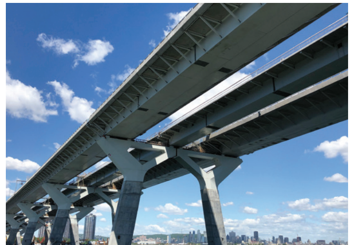
Samuel de Champlain bridge in Montreal
