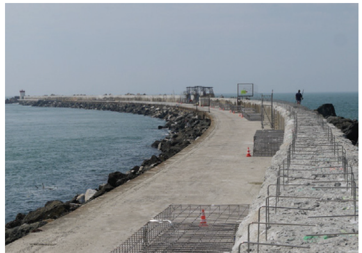
Repair of the Northern Breakwater of the port of Bayonne
